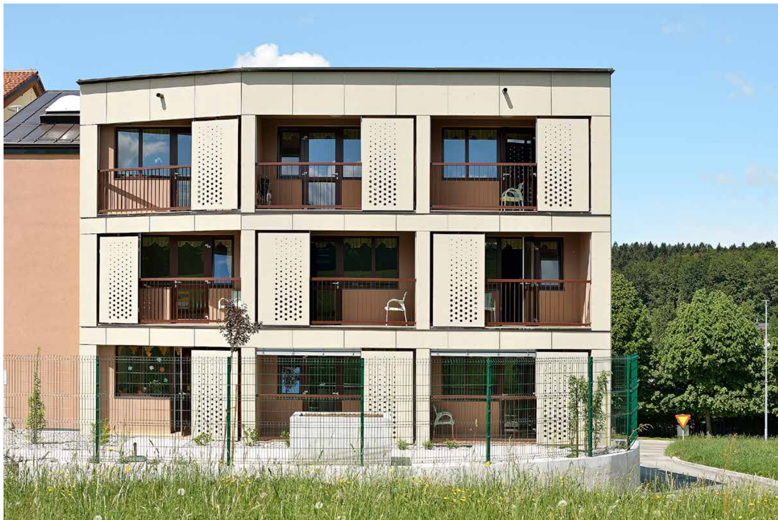
Perforated Swisspearl panels allow dappled light in, whilst affording a sense of privacy.
