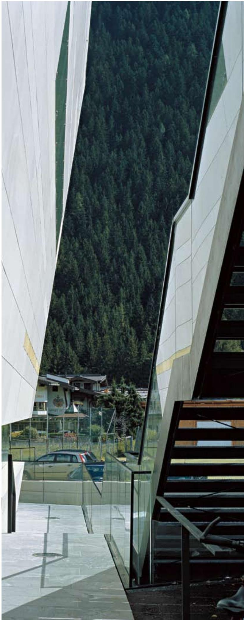
White cement composite panels, large-scale ribbon windows, and narrow lighting strips made of coloured sintered glass enclose the planar, chiselled volume.
