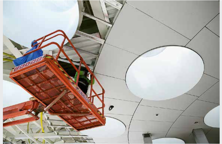
Large skylights pierce through the roof and illuminate the interior. Spirally arranged Swisspearl panels accentuate the circular shape of the roof.
