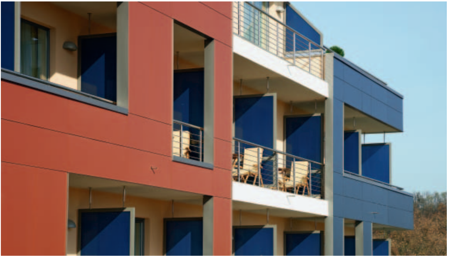
The loggias are constructed of light metal and attached to the edge of the reinforced concrete panels.
