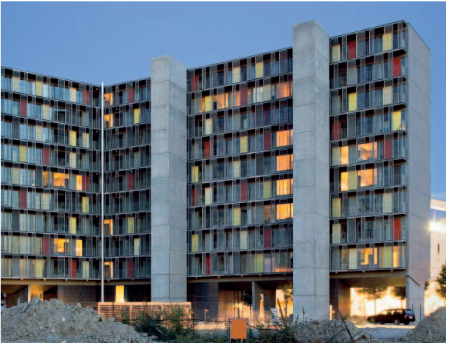
A VARIOUSLY DESIGNED FAÇADE WITH BALCONIES, METAL SCREENS AND CEMENT COMPOSITE PANELS.
